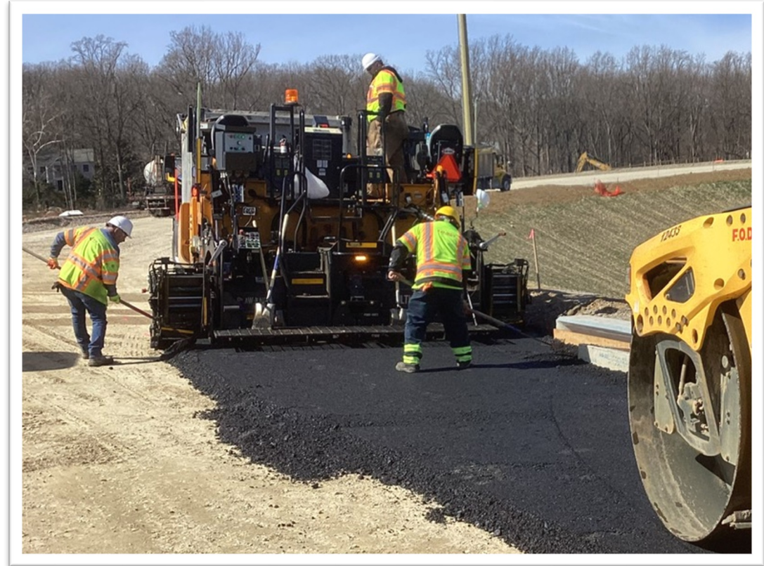
A crew lays down base asphalt for the future GW Parkway to southbound I-495 ramp (March 2024)
