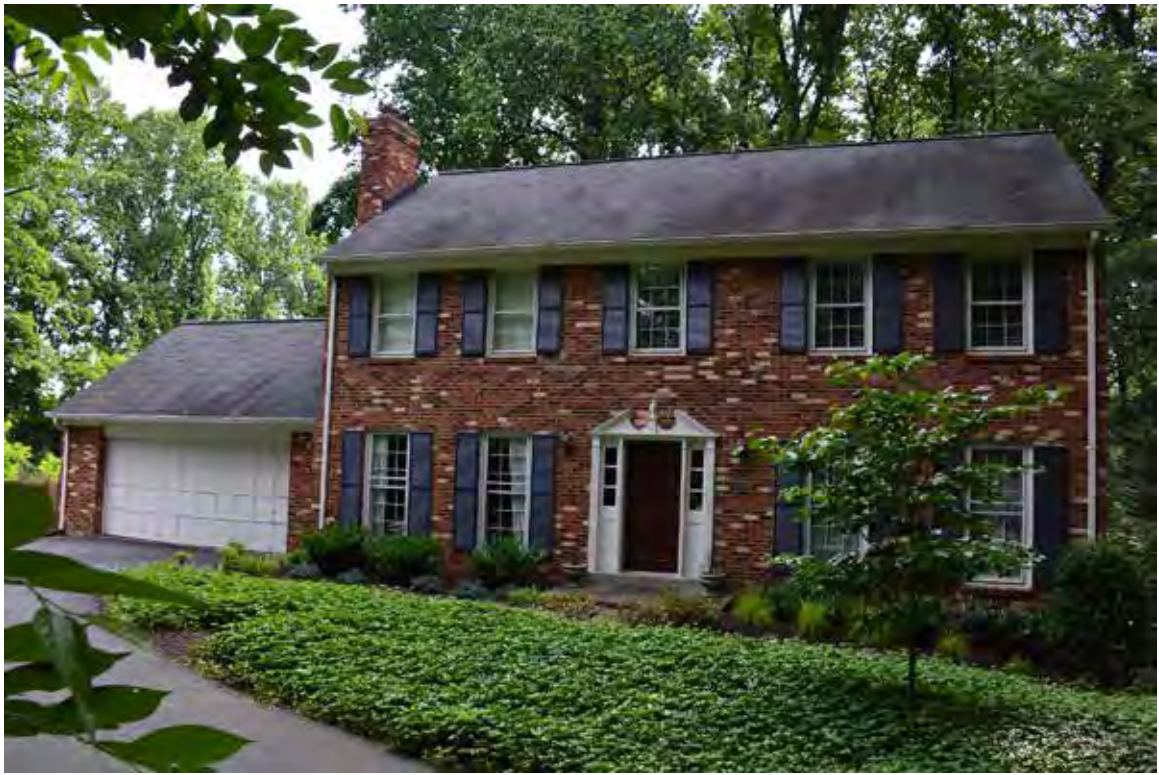
Figure 33. 7048 Arbor Lane (029-6541), house, façade.
