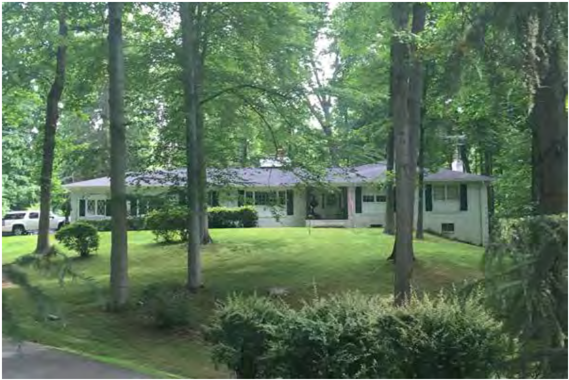
Figure 23. 6706 Lupin Lane (029-6528), house, façade.
