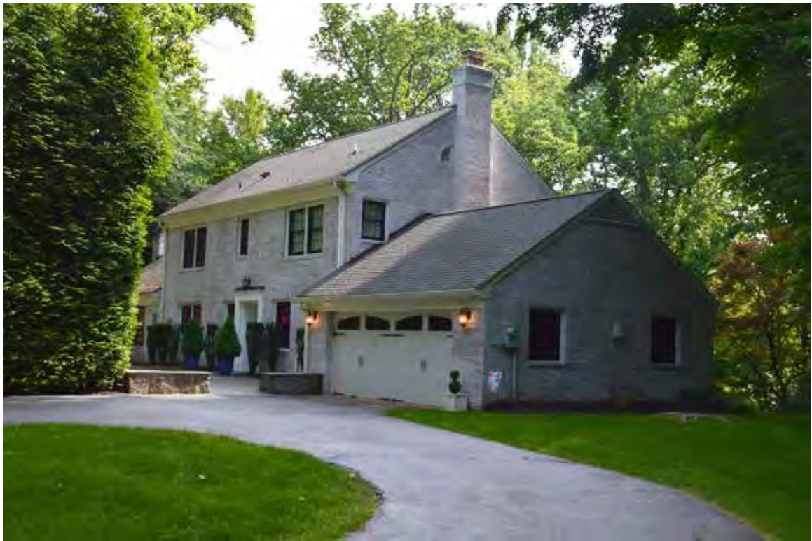
Figure 31. 710 Live Oak Drive (029-6539), house, view north.
