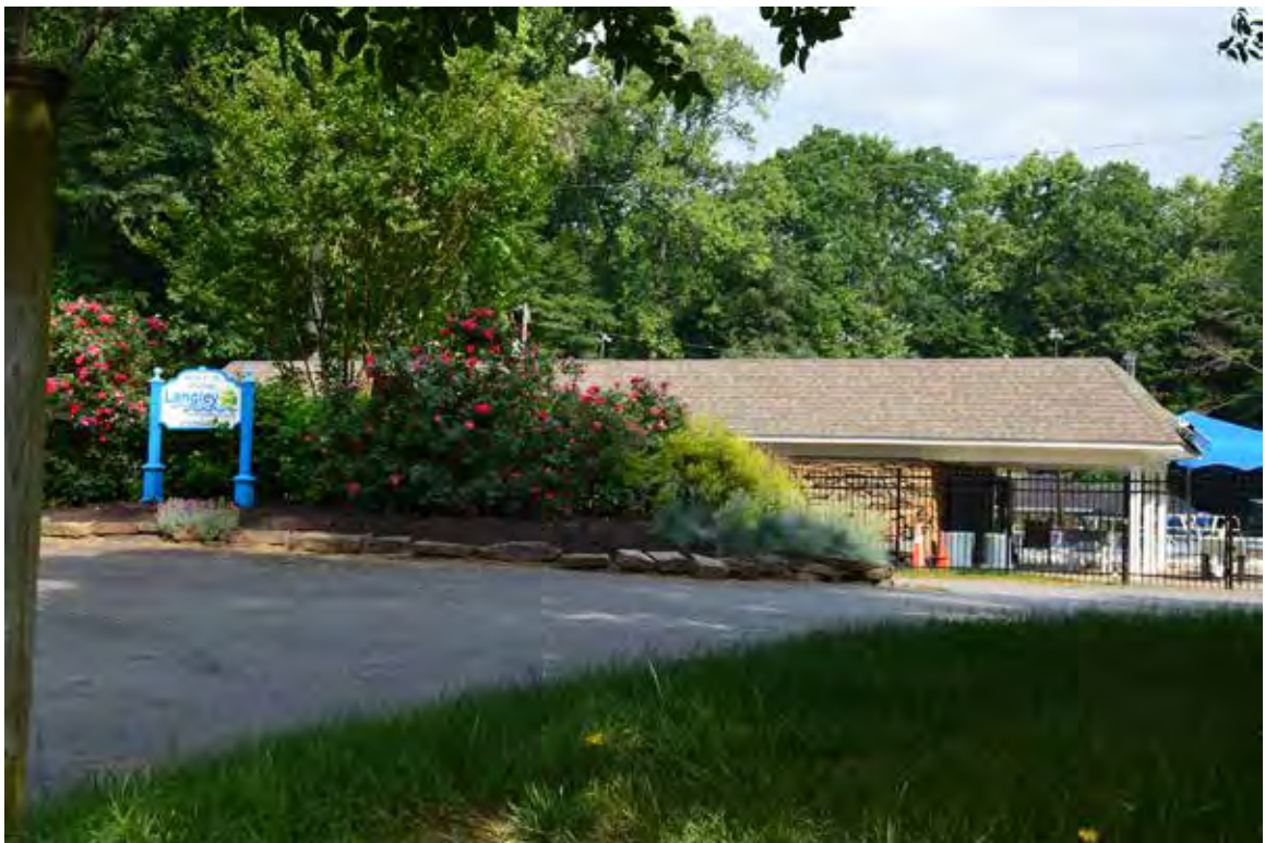
Figure 32. Langley Club, 728 Live Oak Drive (029-6540), entry building, view northwest.
