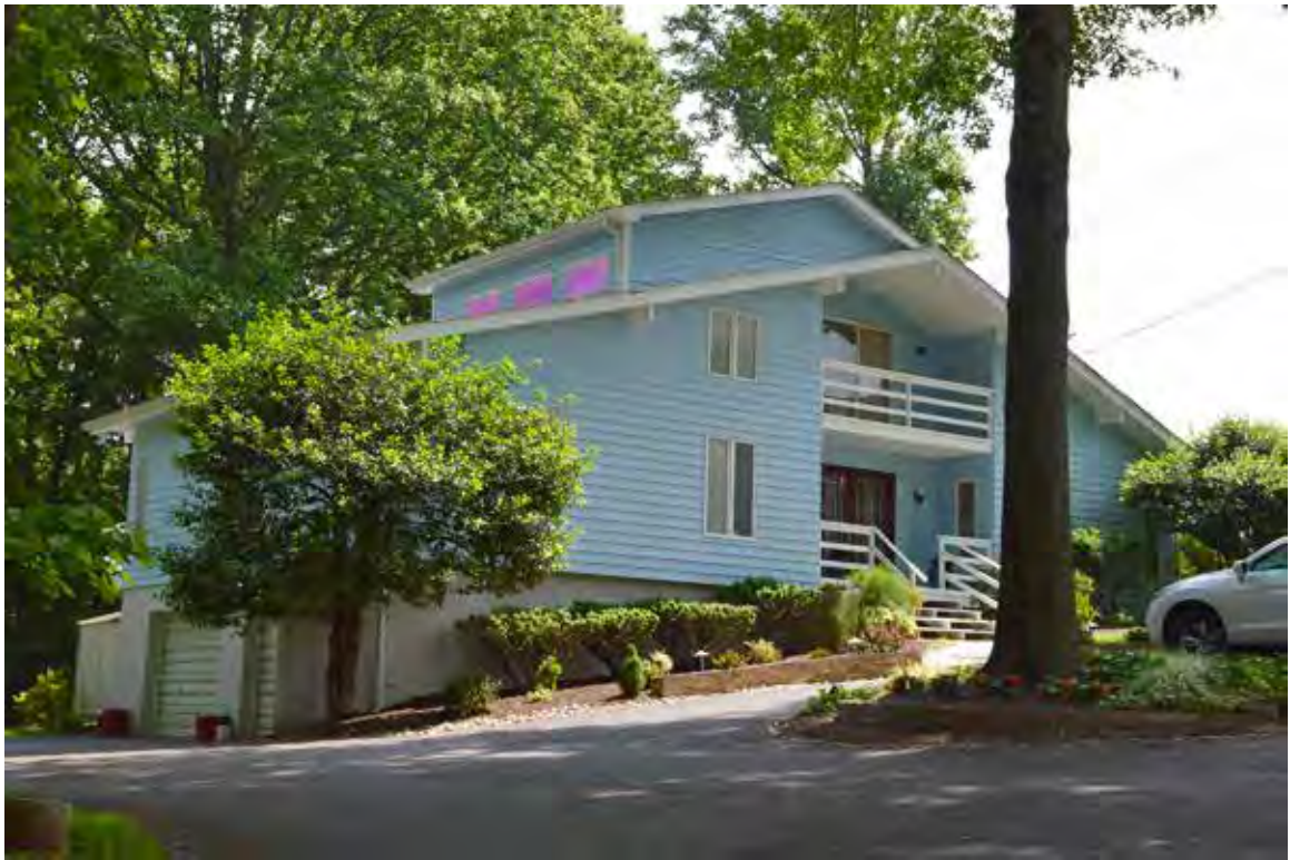
Figure 47. 987 Spencer Road (029-6553), house, view northeast.
