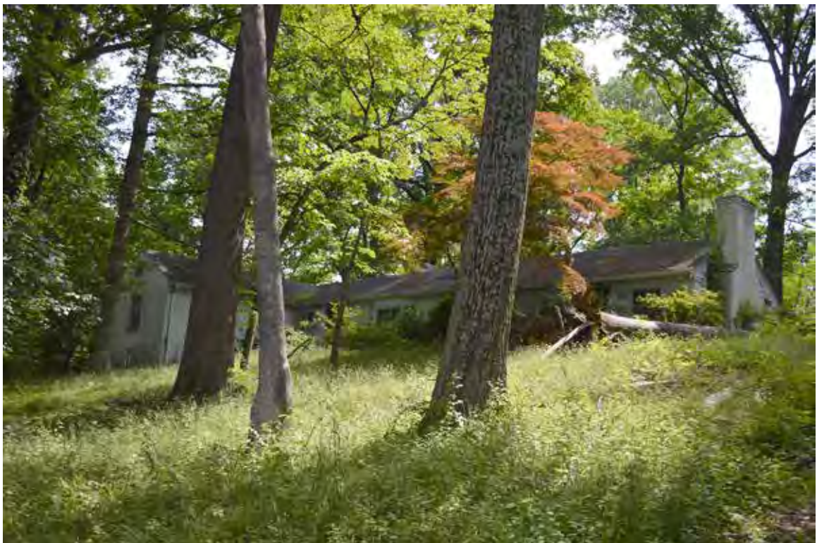
Figure 68. 7448 Dulany Drive (029-6565), house, view northeast.
