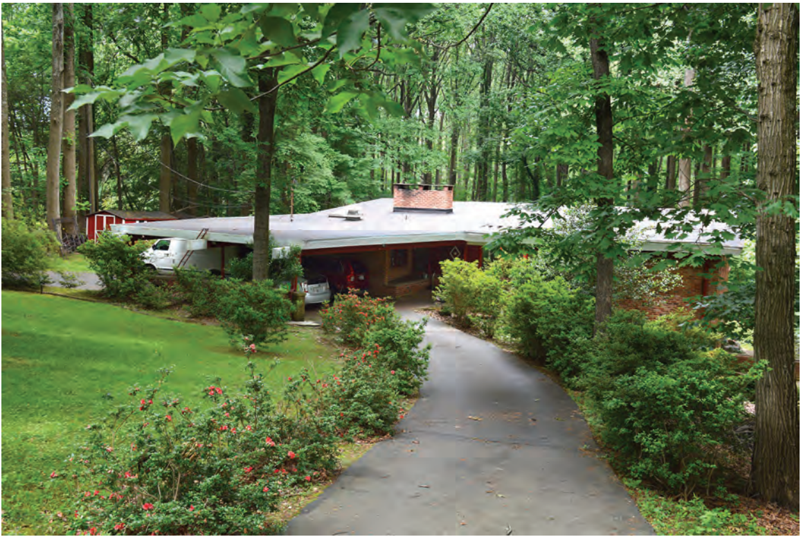
Figure 73. 7421 Dulany Drive (029-6578), house and shed, view south.
