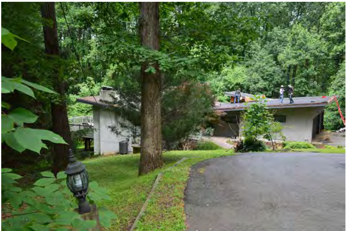
Figure 72. 7425 Dulany Drive (029-6577), house, view southwest.
