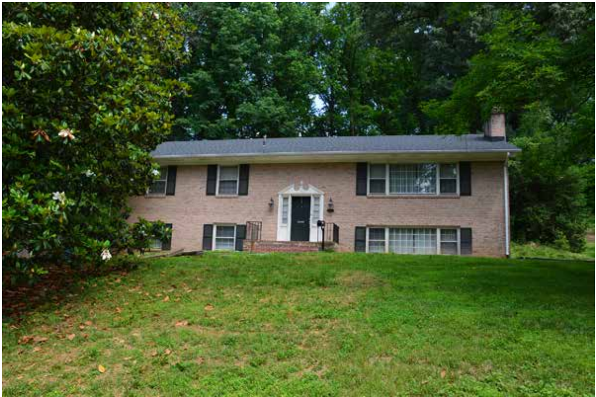
Figure 53. 7404 Churchill Road (029-6558), house, façade.
