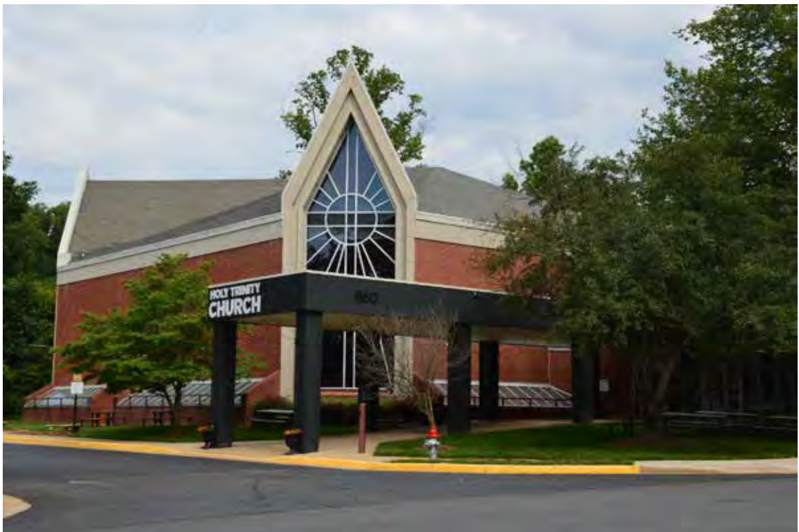
Figure 38. Holy Trinity Church, 850 Balls Hill Road (029-6546), church, entry into 1992 addition.
