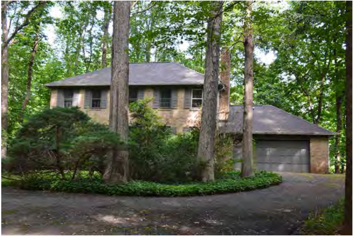
Figure 34. 7050 Arbor Lane (029-6542), house, façade.
