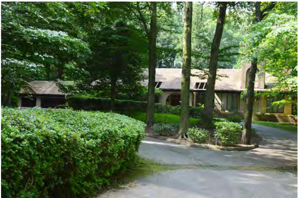
Figure 44. 7321 Georgetown Pike (029-6551), house, façade.
