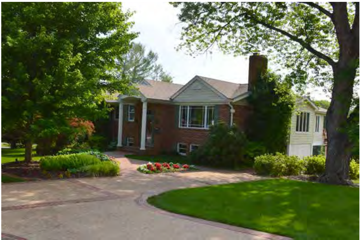
Figure 40. 931 Dead Run Road (029-6547), house, view northeast.
