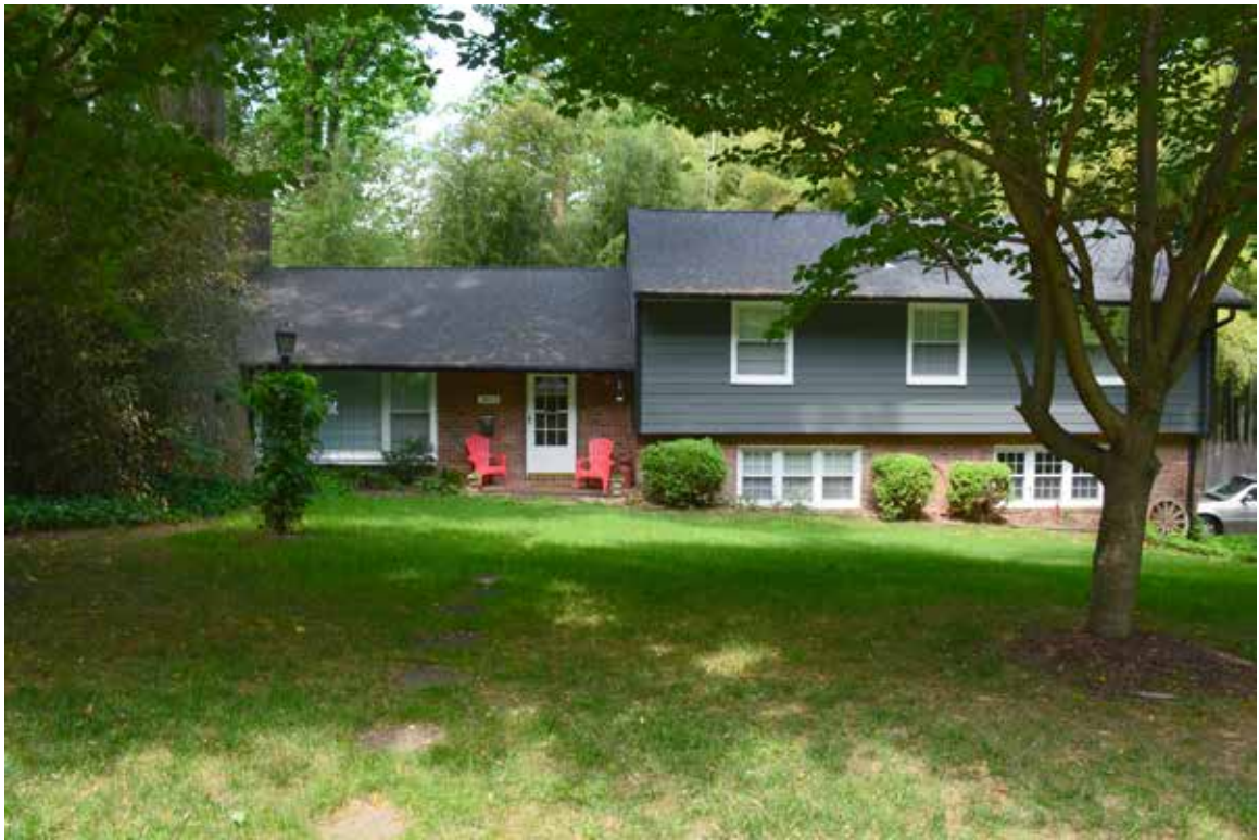
Figure 55. 7412 Churchill Road (029-6560), house, façade.
