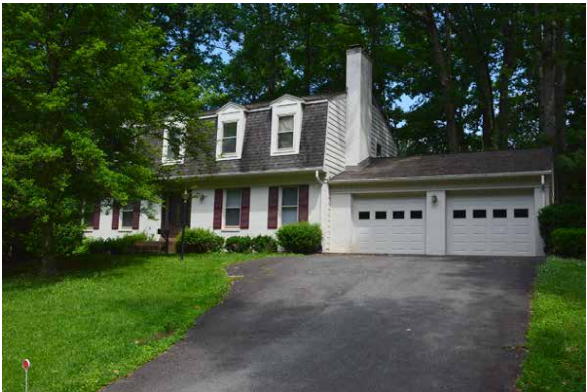
Figure 54. 7408 Churchill Road (029-6559), house, view southwest.
