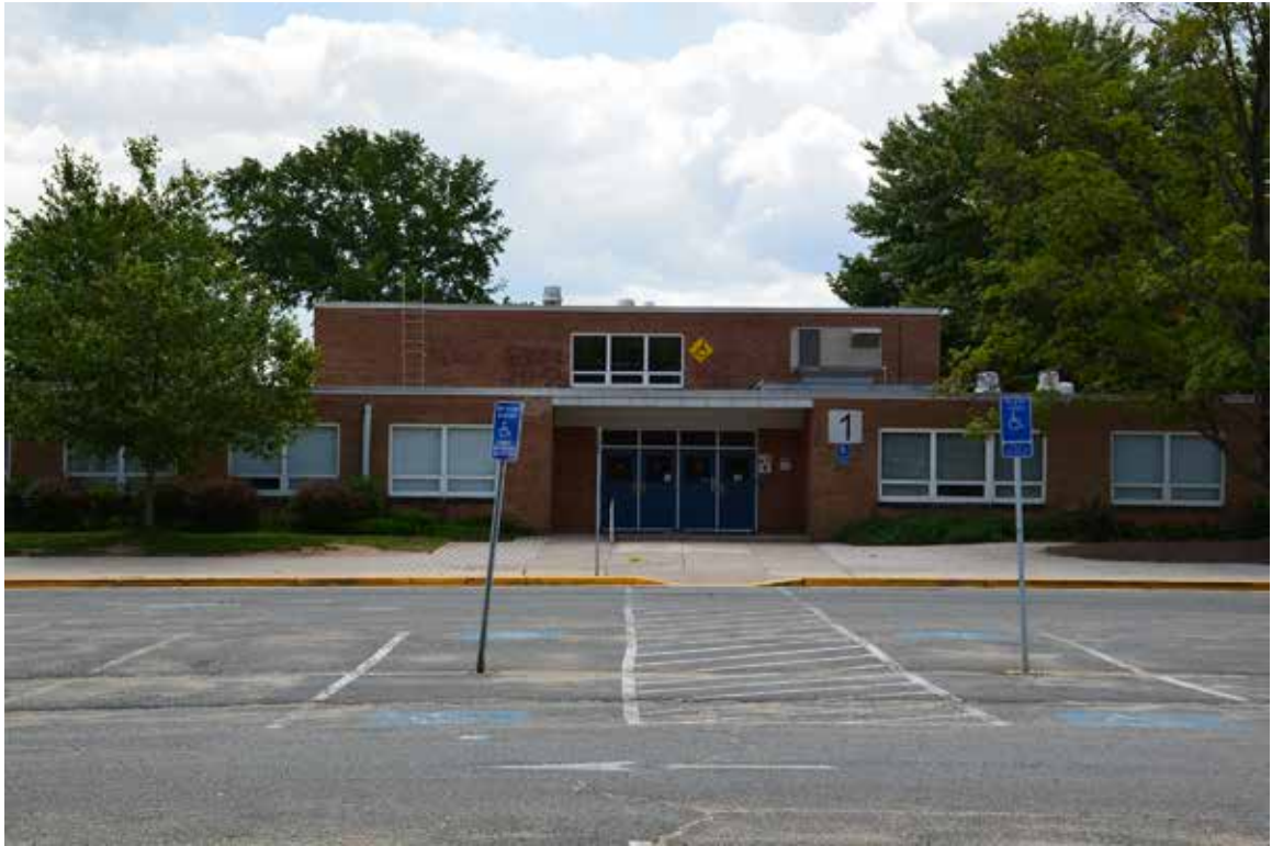
Figure 42. Cooper Middle School, 977 Balls Hill Road (029-6549), school, entry and facade.
