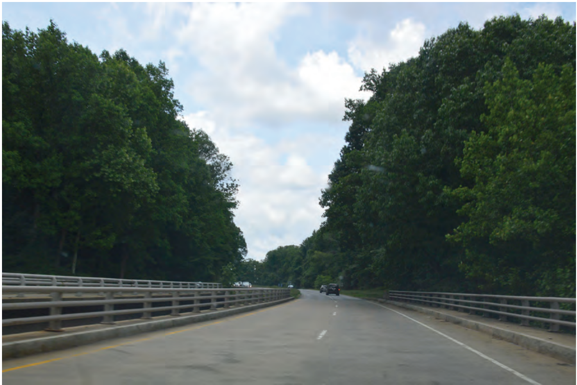
Figure 17. George Washington Memorial Parkway (029-0228), view westbound from bridge over Dead Run.
