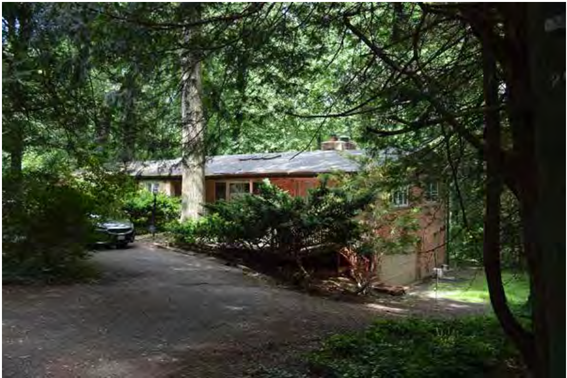
Figure 71. 7433 Dulany Drive (029-6576), house, view southwest.
