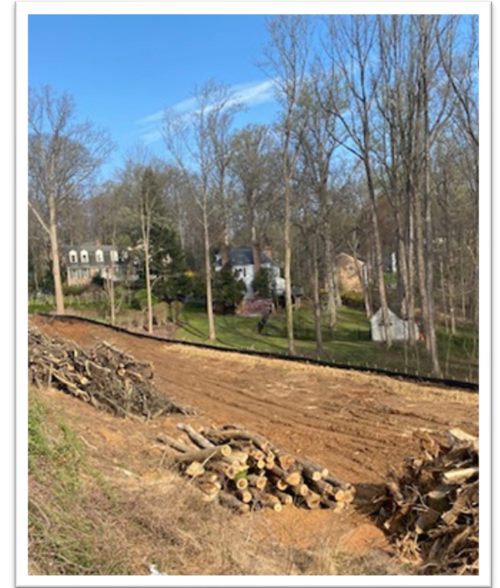
View from Old Dominion Drive (March 2023)
