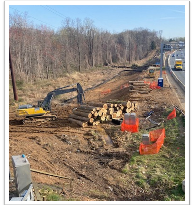
Clearing along southbound Beltway near Old Dominion Drive (March 2023)
