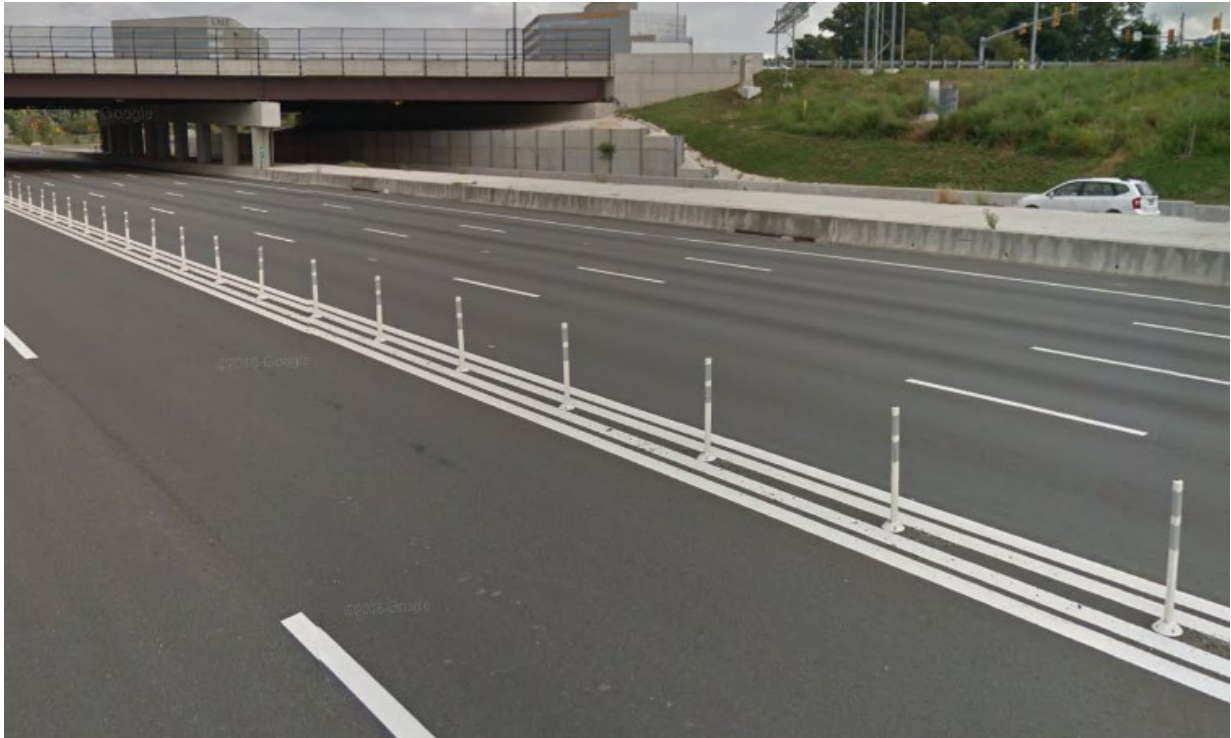
Figure 6-1. Existing Flexible Post Delineators on I-495 Express Lanes
