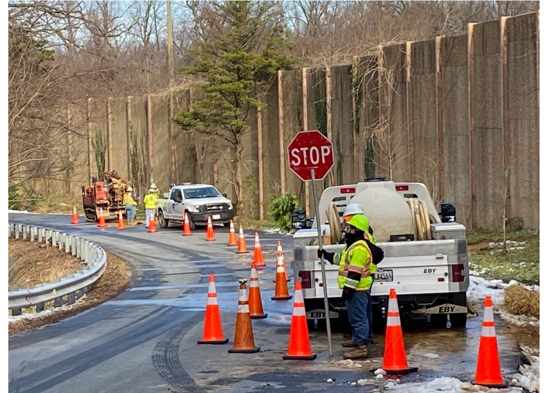
Single-lane traffic operation on Live Oak Drive during January 2022 test boring
