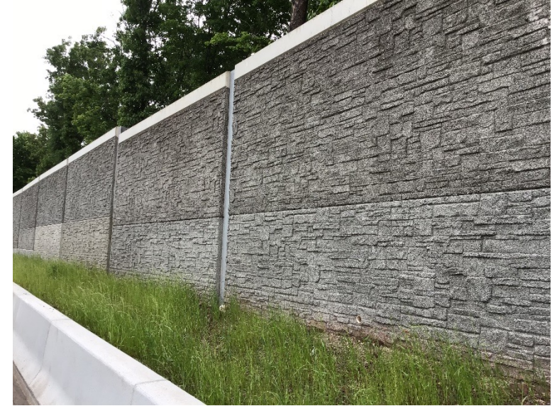
Example of dry stack (simulated stone) noise wall
